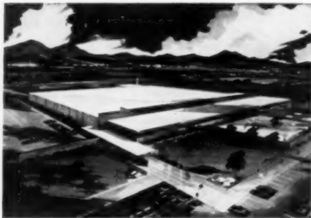
Denver plant now under construction will augment the Division's manufacturing facilities
